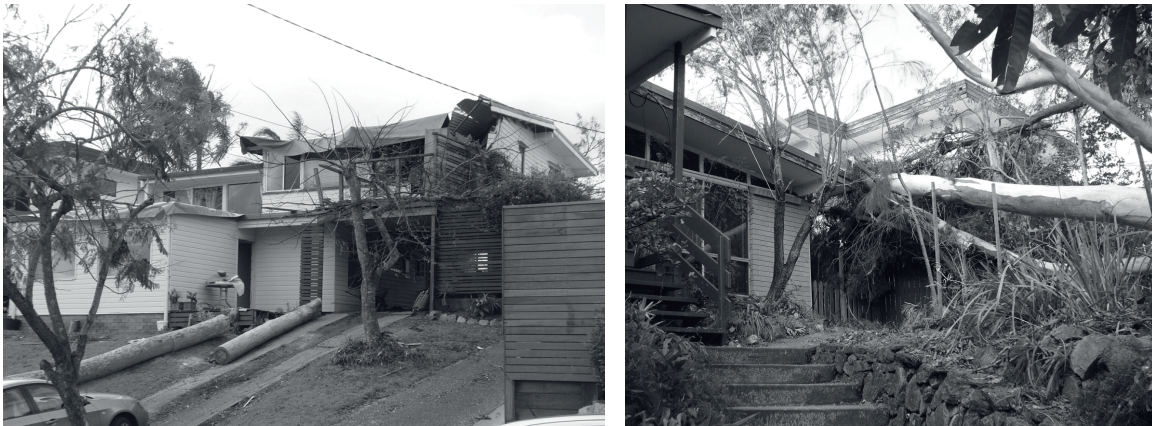
Figure 10: Damage to housing caused by large falling trees in The Gap.
