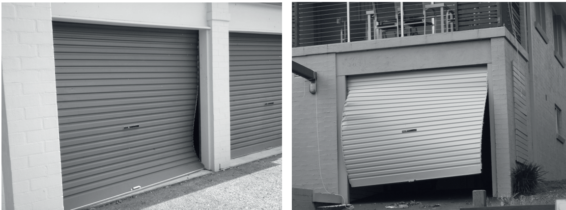
Figure 15: Typical roller door failures.
