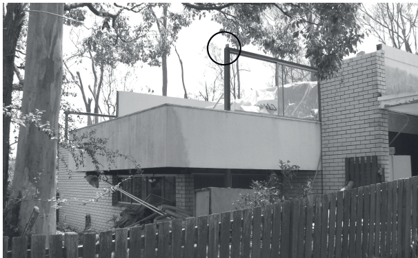
Figure 16: General view of front of house without roof.
