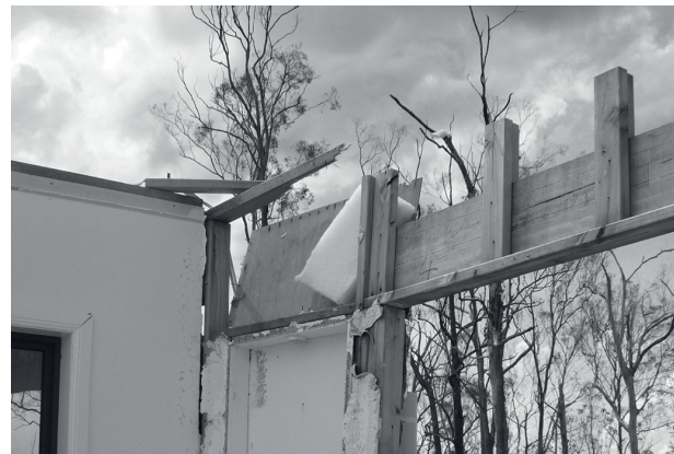
Figure 23: Lintel to back window, held down by ply bracing panel.
