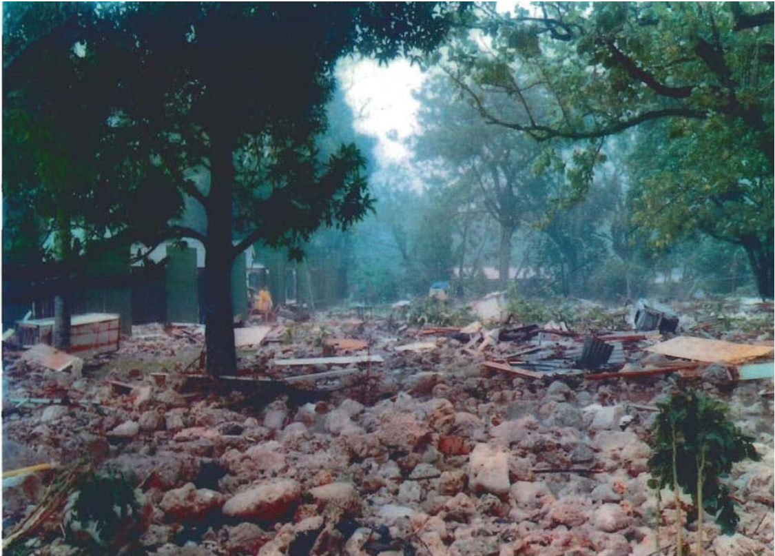
Rubble on higher section of road between Avatiu and Avarua
