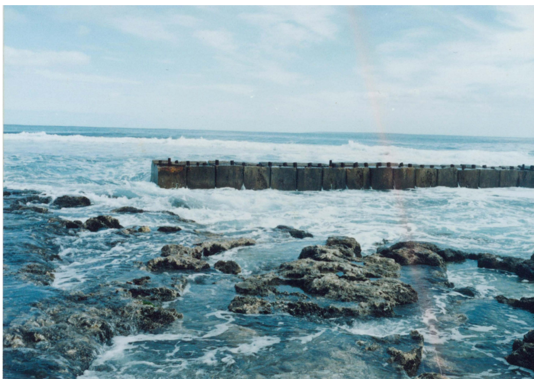
South Breakwater Nafanua Harbour, 'Eua showing flow of reef setup water between end of breakwater and shore. (Closure of this gap raised reef flat water levels by approx 0.4m during normal weather
