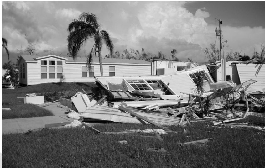
Figure 2. Mobile home damage in Hurricane Charley (2004)
