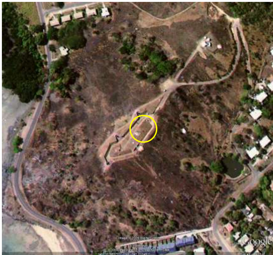
Figure 3-6 Steep site of the former Thursday Island MO wind station. (Google Earth™ images)
