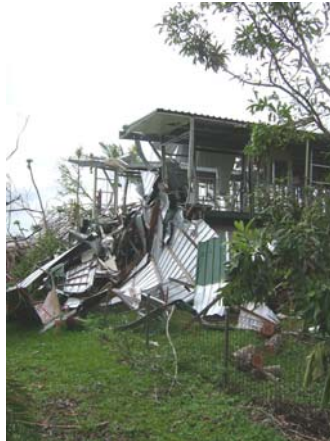
Top: An older house with typical loss of roofing; Bottom: A newer house destroyed by a flying roof, removed from an older house, that had passed over several other low set homes.
